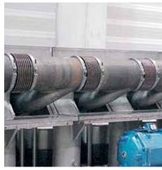
UM type expansion joints installed on an engine system.
