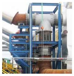
US type expansion joints installed at a flue gas exhaust system at a power plant.
