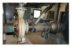
In the pulp production at Stora Enso Skutskär in Sweden, a Sulzer APP Ahlstar pulp pump transports the pulp with black liquor to the washing and bleaching processes. The pump is equipped with an EagleBurgmann **Cartex-DN** with a connected **BestFlow** pressure regulating valve for the optimum supply of buffer water to the seal. Operating conditions:  $p = max. 4.5 \ bar (65.3 \ PSI), t = 66 \ ^{\circ}C (151 \ ^{\circ}F), n = 956 \ min^{-1}.$
