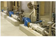
At Iggesund Paperboard, Workington, UK, eccentric screw pumps with MG1S50 type cartridge seals are operating reliably in the coating plant. Medium: Coating color, p3 = 4 bar (58 PSI), t3 = 40 °C (104 °F), n = 850 min  $^{-1}$ .
