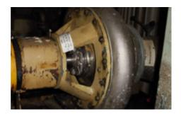
At Stora Enso Kvarnsveden, Sweden, several pumps of the paper machines are sealed with EagleBurgmann **MA251**. Medium: pulp with a solids content up to 1.5 %. Operating conditions: p=2 bar (29 PSI), t=30 °C ... 40 °C (86 °F ... 104 °F), n=1,490 min 1.
