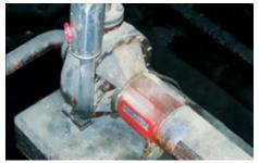
At the UPM Pietarsaari pulp mill in Finland, a Sulzer APP 23 pump is sealed with an EagleBurgmann Mtex-TN. This cartridge version of the metal bellows seal is particularly suitable for highly viscous media at low temperatures. Operating conditions: p = 1 bar (15 PSI), t = 120 °C (248 °F),
