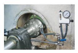
Chest agitators at Sappi in Lanaken/Belgium were retrofitted to EagleBurgmann **HGH** type semi-split mechanical seals. Since then, product leakage has been drastically reduced and plant availability has noticeably increased. Operating conditions:  $p = 0.5 \text{ bar } (7.25 \text{ PSI}), t = 20 ^{\circ}\text{C} \dots 40 ^{\circ}\text{C}$  $(68 \, ^{\circ}F \dots 104 \, ^{\circ}F), n = 300 \, min^{-1}.$
