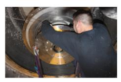
A Pulpex-S/135-00 is installed in a sorter at the Sappi paper mill in Lanaken/Belgium. The mechanical seal runs in a continuous process in pulp preparation. Operating conditions: p = 3.5 bar (51 PSI),  $t = 80 \, ^{\circ}\text{C} (176 \, ^{\circ}\text{F}), \, n = 800 \, \text{min}^{-1}. \, \text{Medium: pulp.}$
