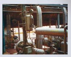
Most of these applications are based on dual mechanical seals. They are pressurized by a central buffer pressure system. Both demineralized water in one section and clean process water for the rest of the plant is used as buffer medium (ring main).
